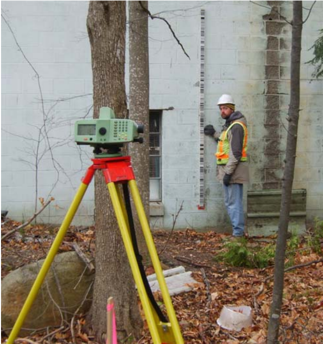
Checking target on building for settlement with a digital level.
