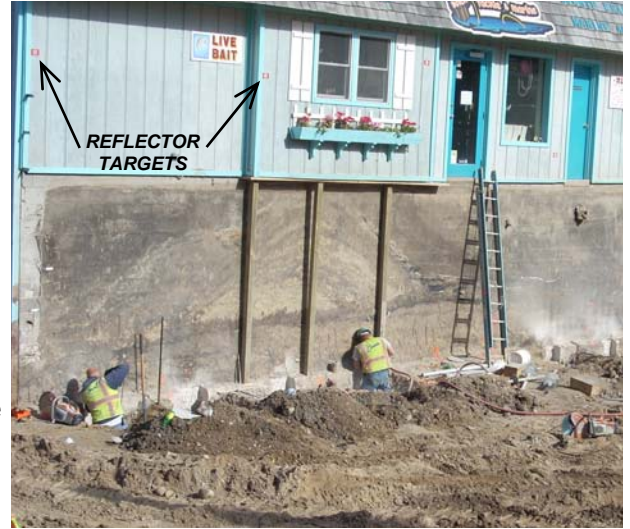
Installation of underpinning system. Note targets attached to building siding.
