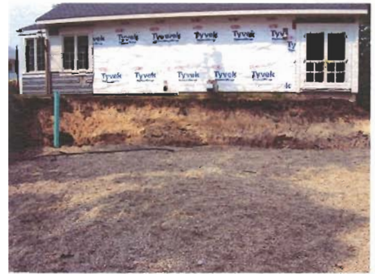
Residence under construction in area of possible soft soils
