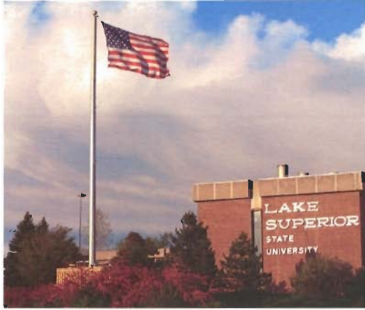
Telecommunication antennas are concealed within the flagpole at Lake Superior State University
