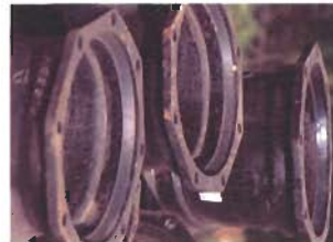
Mechanical Joint Ductile Iron Water Main
